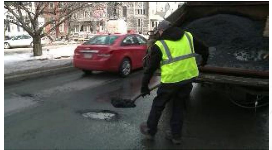
Pothole repair
